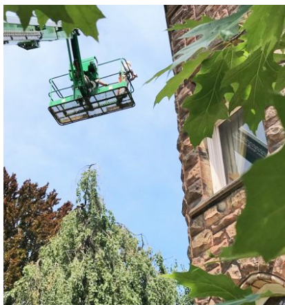
Inspection of roof by slate expert Joseph Jenkins
